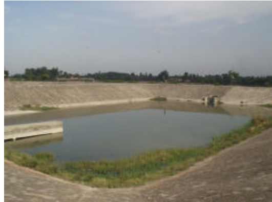
Existing Sewerage Plant A
