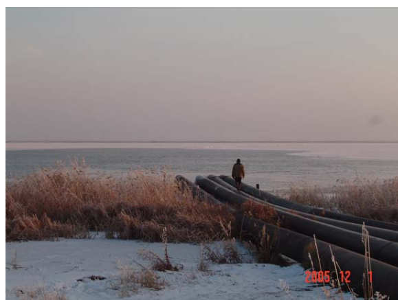
Drain outlet of wastewater treatment plant in the suburb of Astana City (Treated water to be discharged to reservoir)
