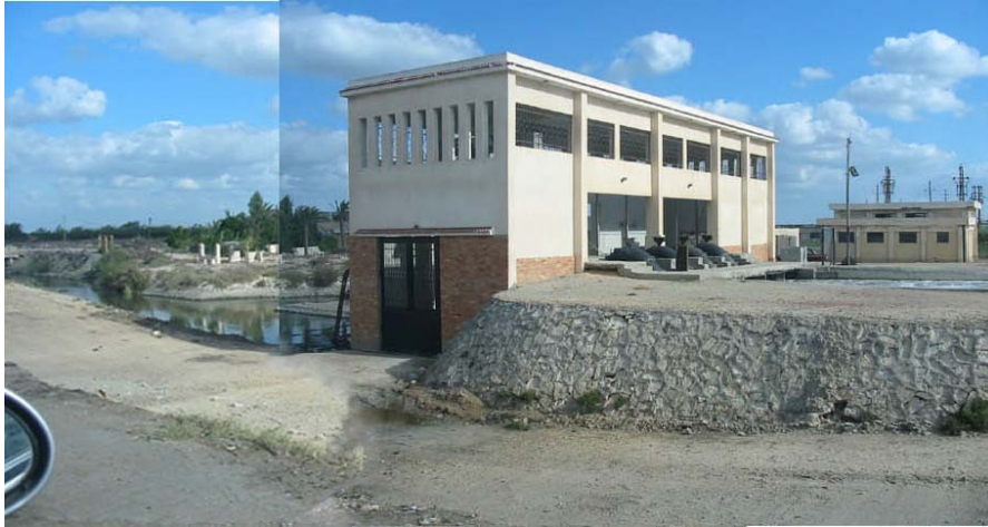
Photo 5.17: Pump Station at Alexandria
