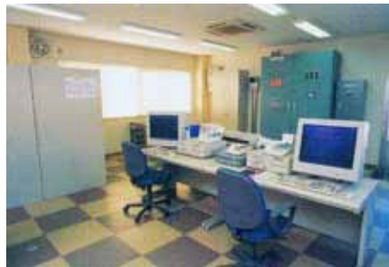
Control Room and Plant Operation
