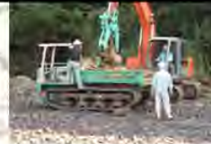
Cleaning by heavy machinery
