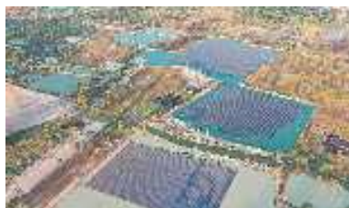
Floating Solar PV, TSB Co., Ltd., Thailand
