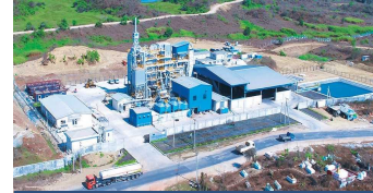
Waste to Energy Plant, JFE engineering, Myanmar
