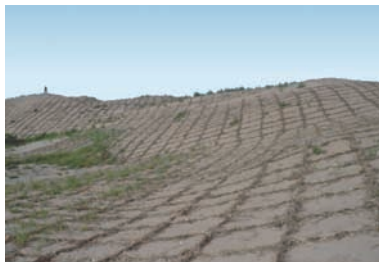
Photo 2 Straw checkerboards
