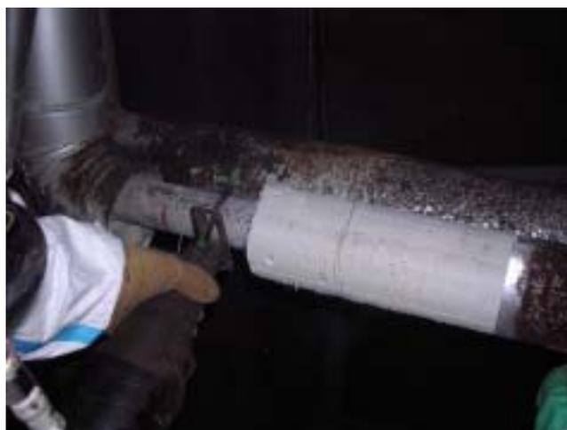
図 4-4-6 配管露出・切断例
